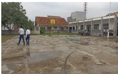
Picture 3. The condition of SMPN 15 in Building 2
